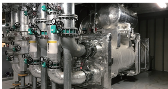
Double-bundled centrifugal refrigerator
